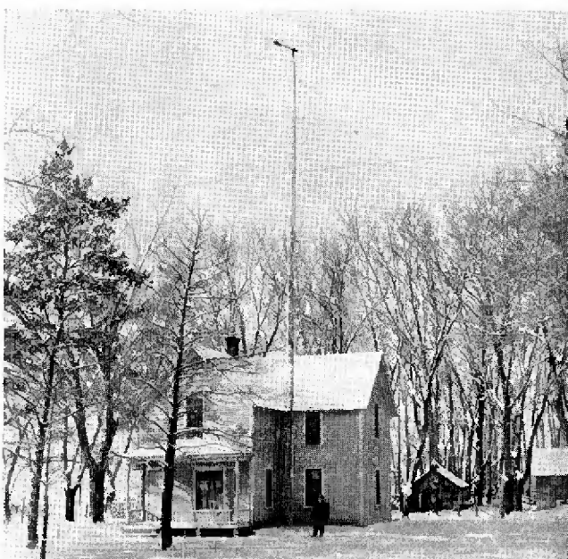
A Dakota farm home, wired for five lights and radio. 400 ampere, glass jar type battery used. A high mast installation made this sale possible
